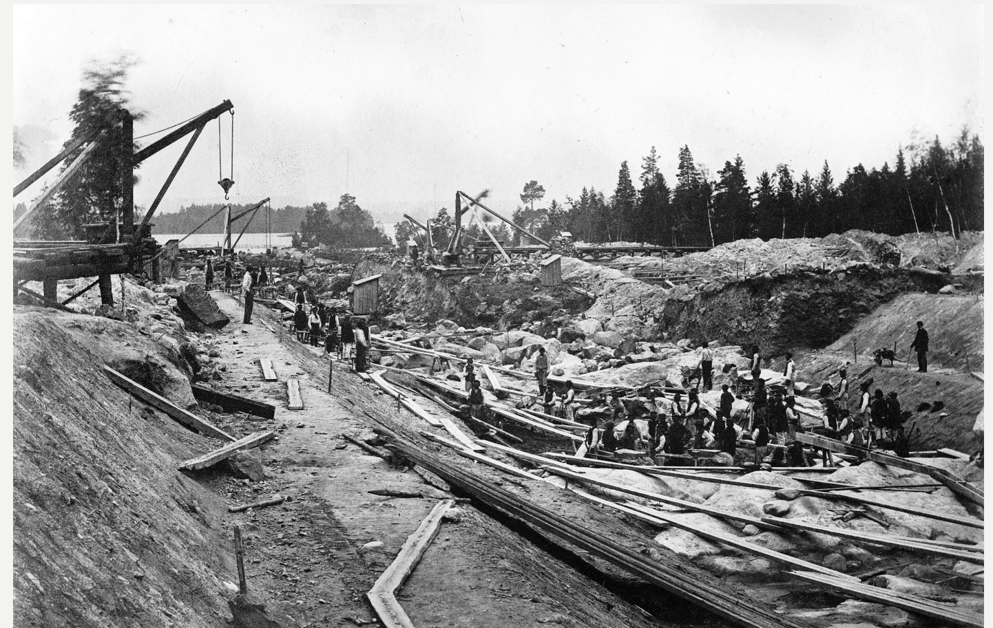
Construction of the Taipale Channel - Image Credit 8
